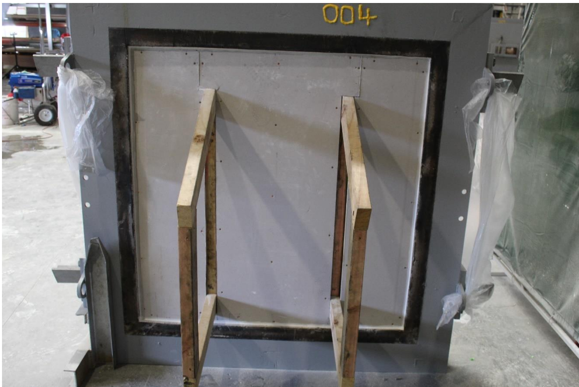
Fig.5 – Unexposed face prior to fire stopping application
